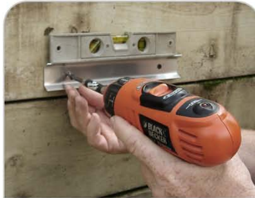
Step 2: Screw in proper screws, making sure to keep bracket level
