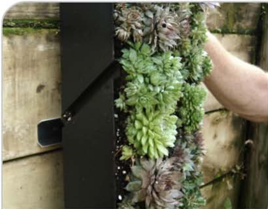
Step 4: Carefully rest Vertical Planter on bracket, making sure it's secure
