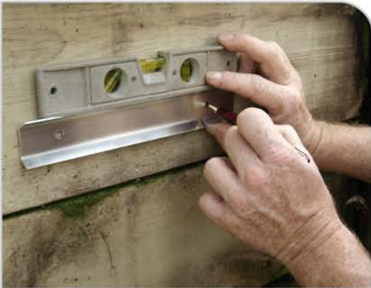
Step 1: Mark holes for the mounting bracket, making sure to keep bracket level
