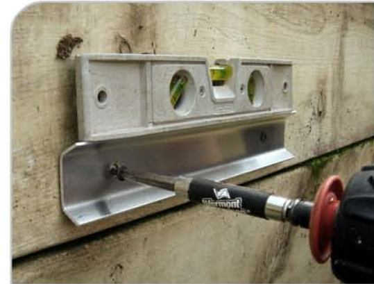
Step 3: Double check level
